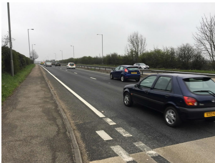
Figure 10 – A27 Upper Brighton Road at the junction with Church Lane looking east
