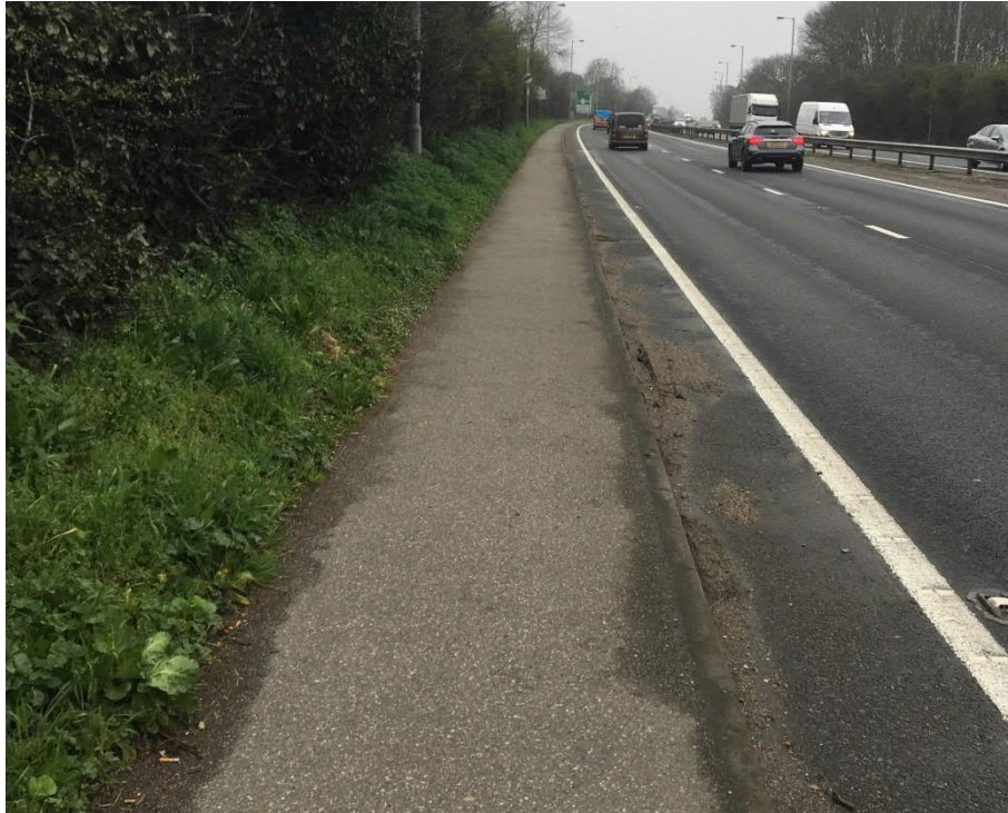
Figure 11 – Footway on the A27 Upper Brighton Road looking east
