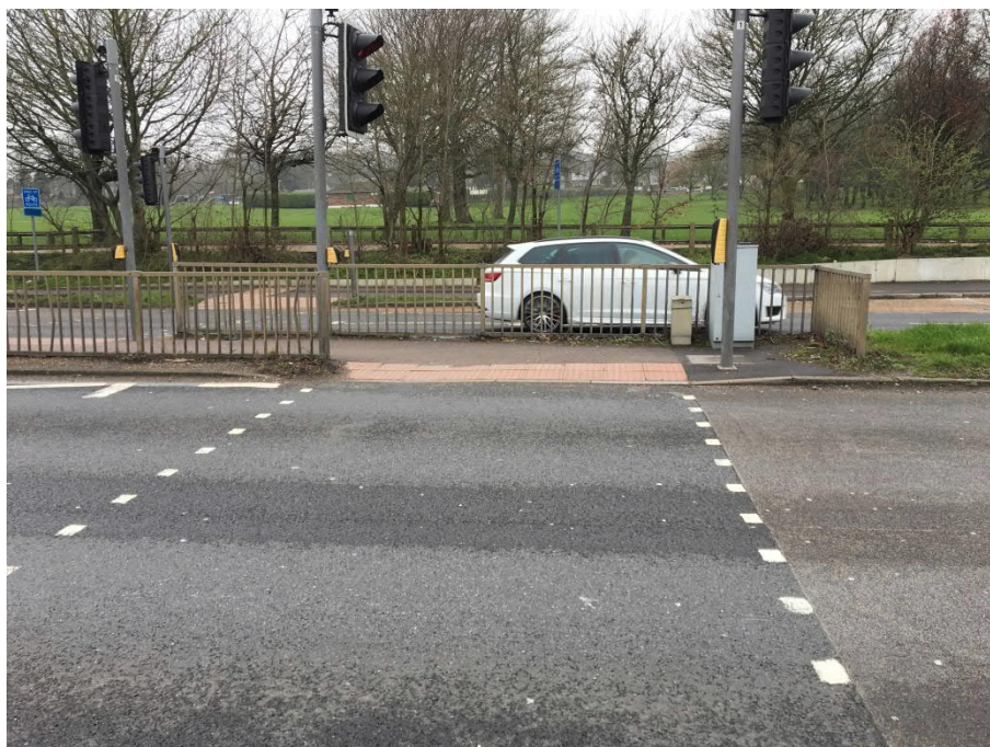
Figure 20 – Toucan crossing on the A27 Old Shoreham Road looking north.
