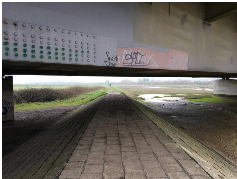
Figure 27 – Footpath 2049 under the A27 Shoreham Bypass looking north
