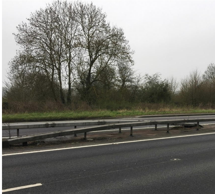
Figure 14 – Central reservation at uncontrolled crossing on A27 Upper Brighton Road near to the junction with Church Lane looking south.
