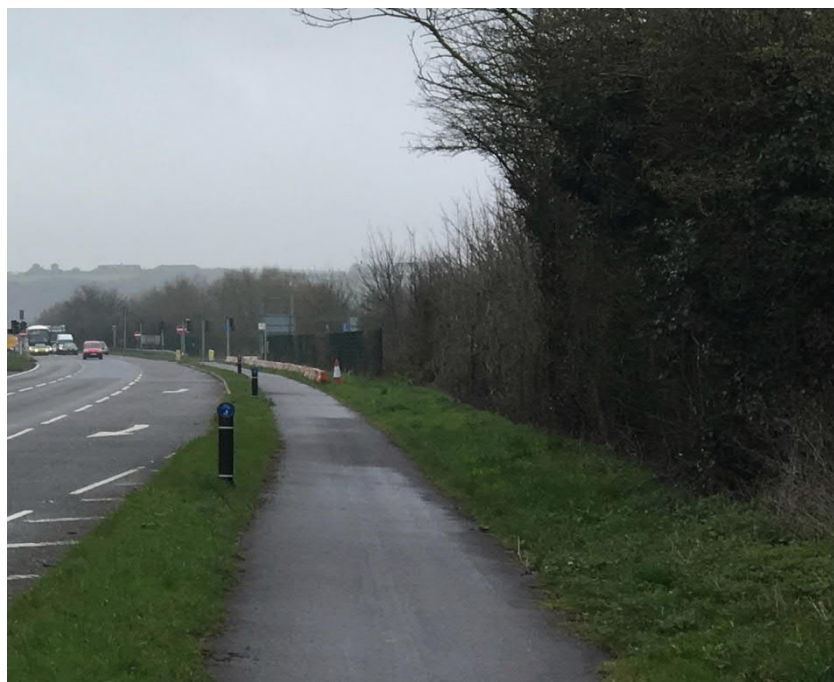
Figure 23 – Bollard mounted signage indicating the shared use path opposite the A27 Old Shoreham Road looking east
